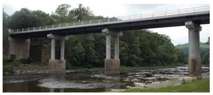
The project involved refurbishing a bridge over the environmentally sensitive River Wye while keeping the bridge open for people cycling or on foot. The client, Powys County Council, and Natural Resources Wales (NRW) had planned the use of hydrodemolition to remove the bridge's existing concrete, but Dawnus, the main contractor, believed this presented a serious environmental risk.
